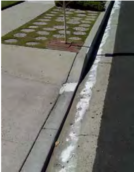
Evidence of an illicit discharge
