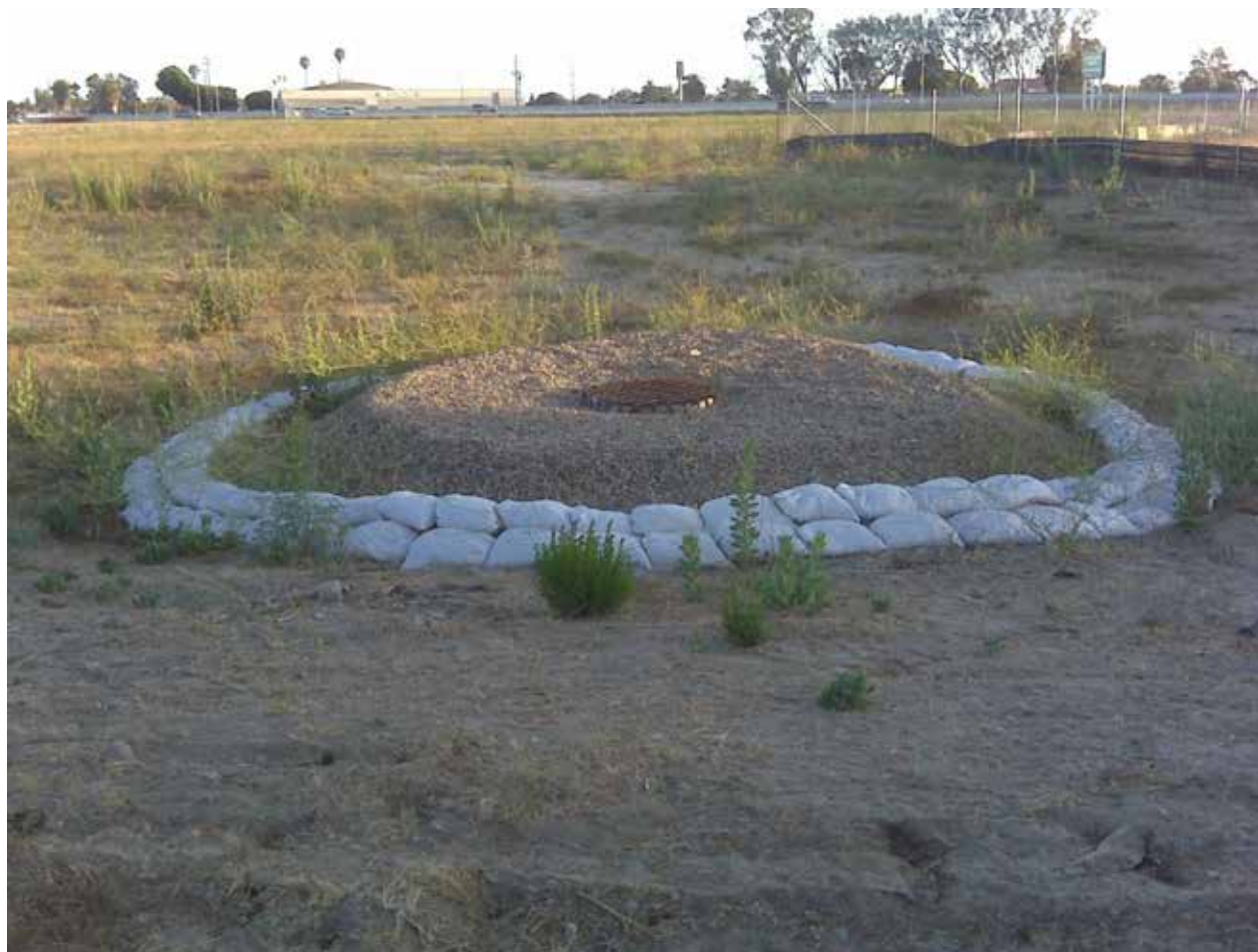
Storm drain protection during construction
