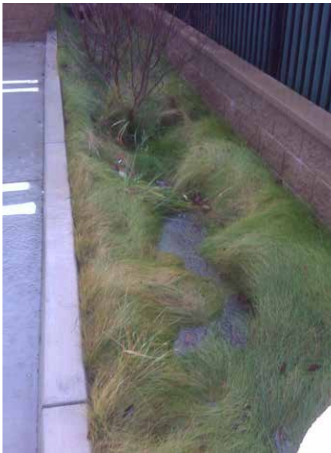
Low Impact Development infiltration BMP
