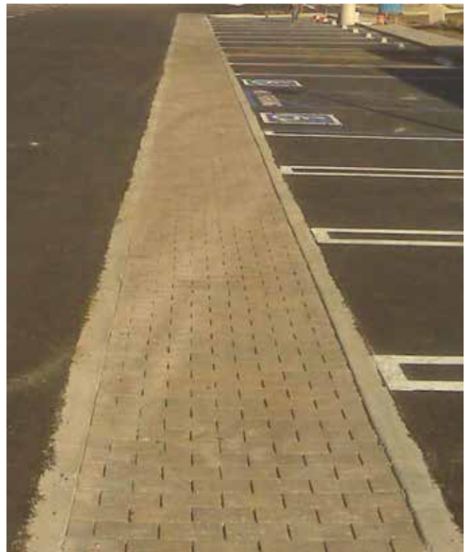
Pervious ribbon gutter in a parking lot
