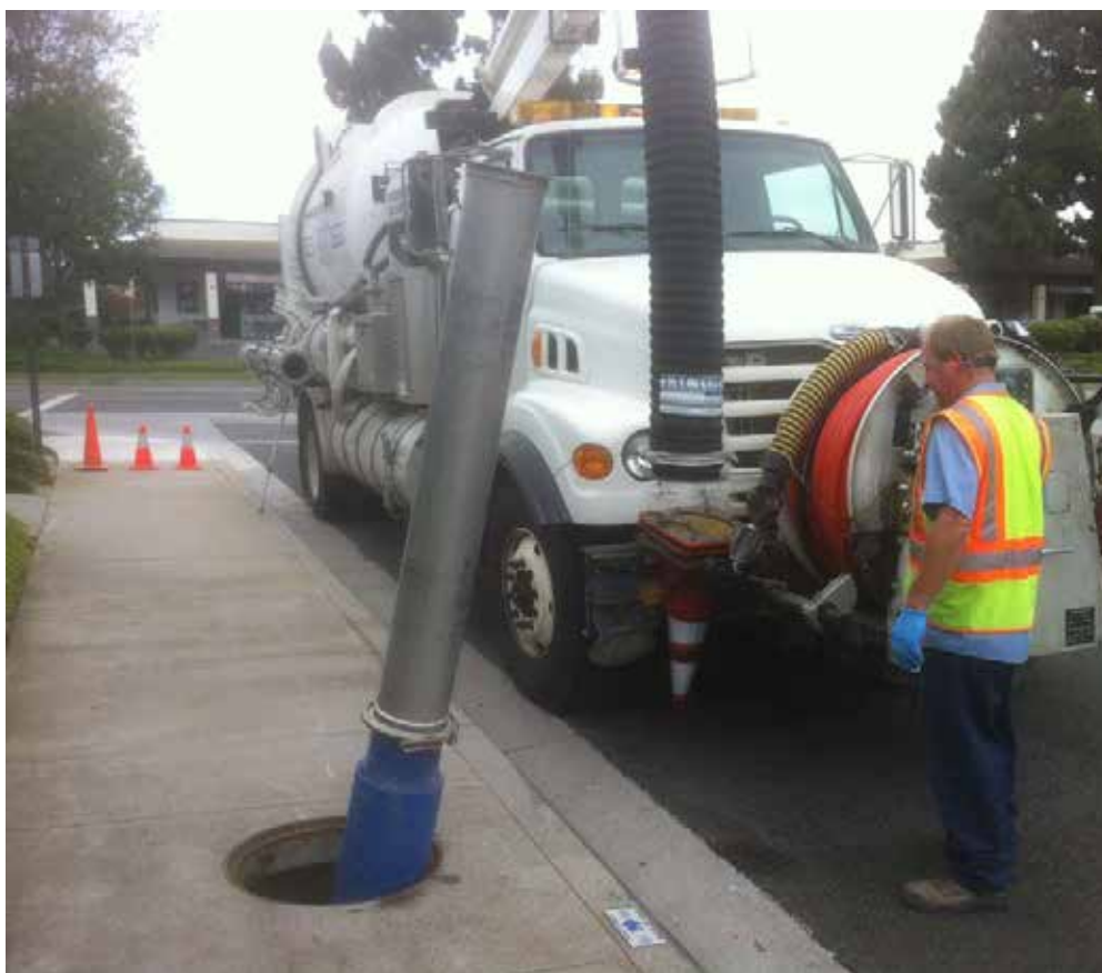
Catch Basin Cleaning Using a Vacuum Truck
